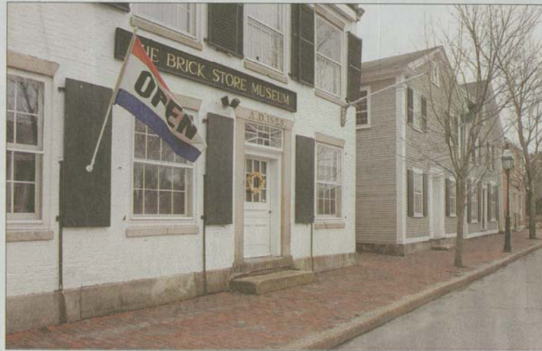
The Brick Store Museum in Kennebunk has received $100,000 to launch a capital campaign for repairs to the museum's buildings, some of which are close to 200 years old. Staff photos by Gregory Rec
